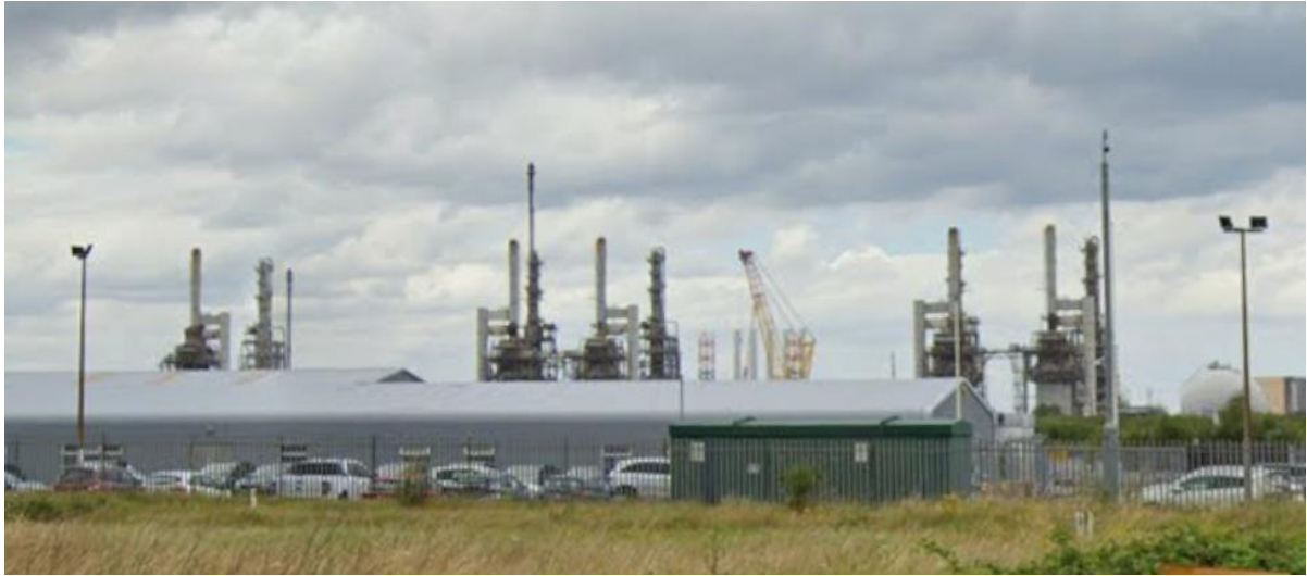
Inset 3.4 Car park areas illuminated from 8M column with angled floodlights on existing site for KD Pharma UK within the new proposed area (image source: Googlemaps Street View)
