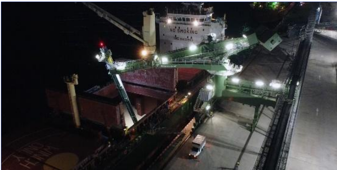
Inset 5.12 CSU lighting example
