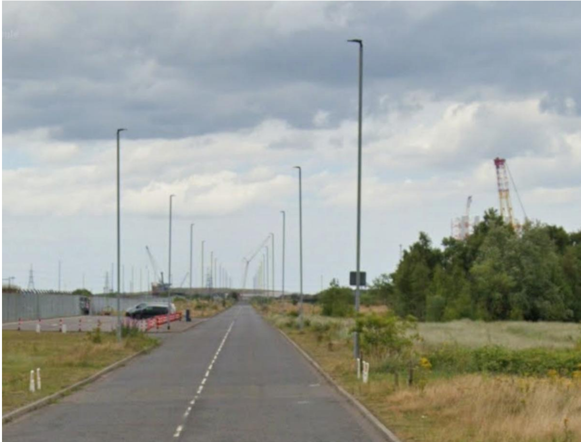
Inset 3.5 Road and access road lighting (image source: Googlemaps Street View)
